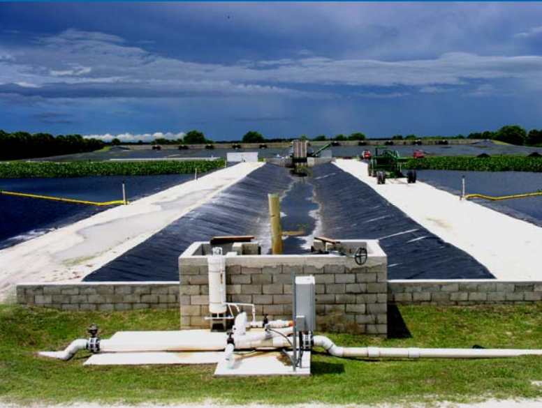
Prototype water hyacinth and algal turf “scrubber” for nutrient removal in Everglades watershed.
