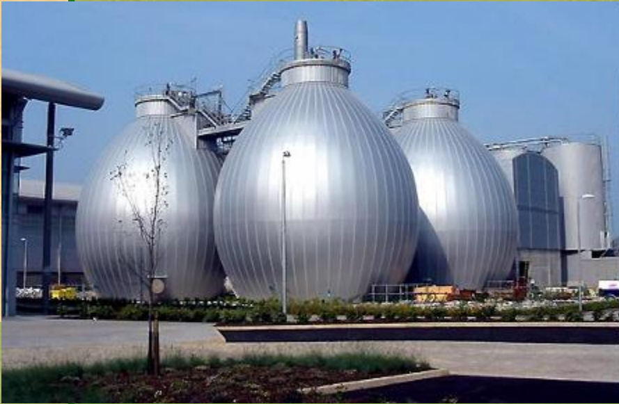
Reading Sewage Treatment Works, Reading, United Kingdom
