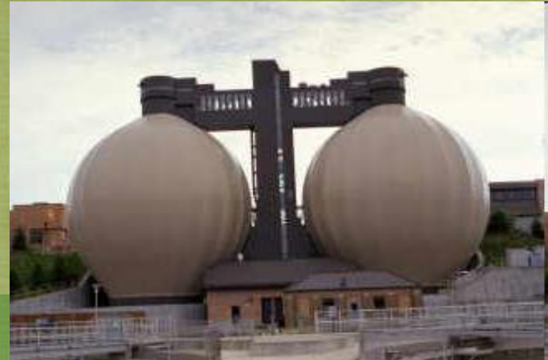
Appleton Wastewater Treatment Plant, Appleton, Wisconsin
