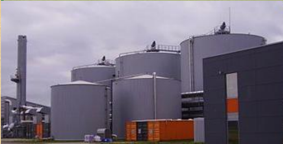
Lübek mechanical biological treatment plant, Germany
