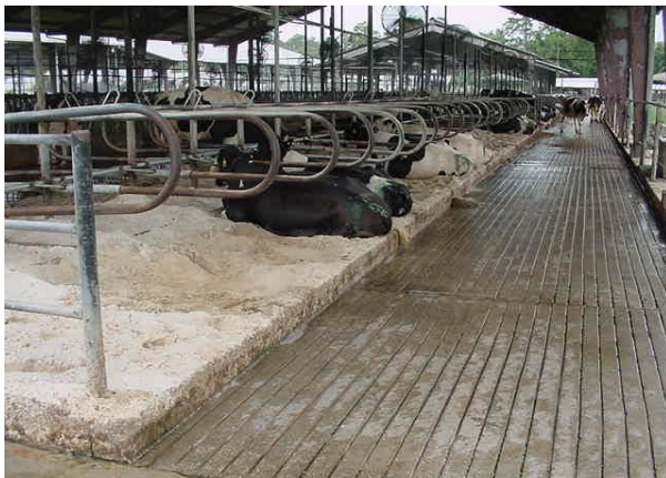
Figure 1: Hydraulically flushed alley.
