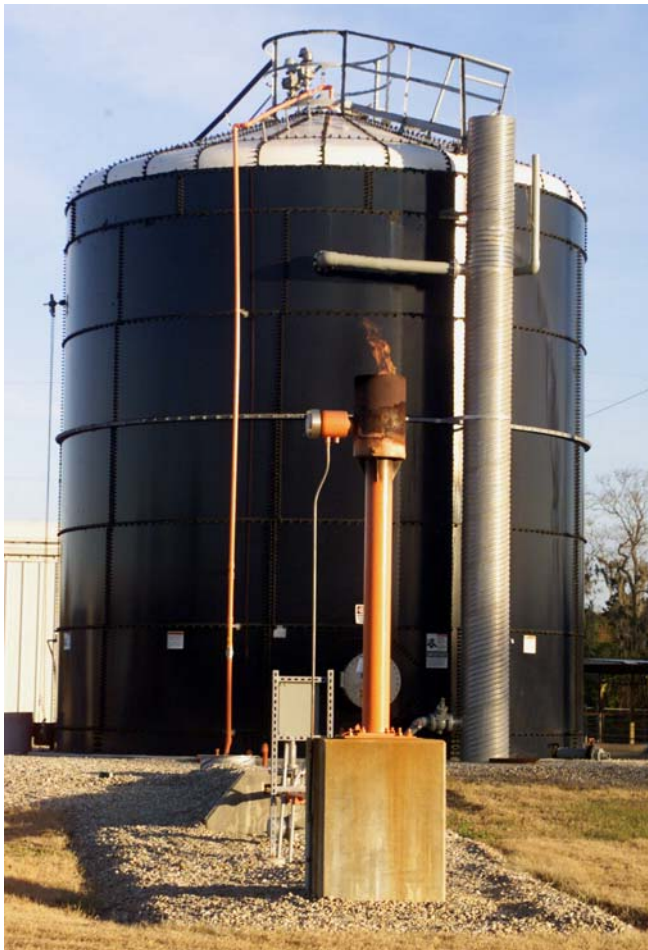
Figure 3: Fixed-Film Anaerobic Digester.
