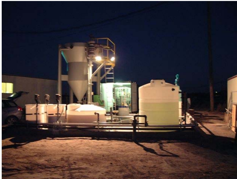
Test Plant for removal of contaminants from acidic Wastewater – Tampa, Florida.
